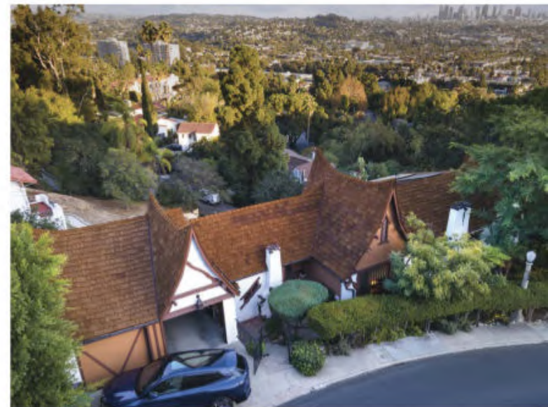
ABOVE The finished roof (solar panels are on the back), with the downtown LA skyline in the distance. TOP The CeDUR shingles are made from over four dozen molds taken of real wood shingles, giving the material exceptional realism.
