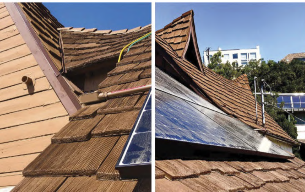
LEFT Photos taken during installation show staggered butts; bending for serpentine curves wasn't necessary on this roof.
