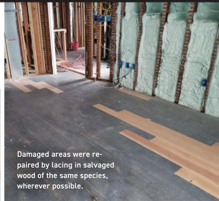
LEFT A sample of the 1" thick vertical-grain Douglas fir that runs throughout the house. The owner was able to use scraps from boards that had to be replaced to make repairs in other locations. BELOW Electrical lines ran under the patch.
