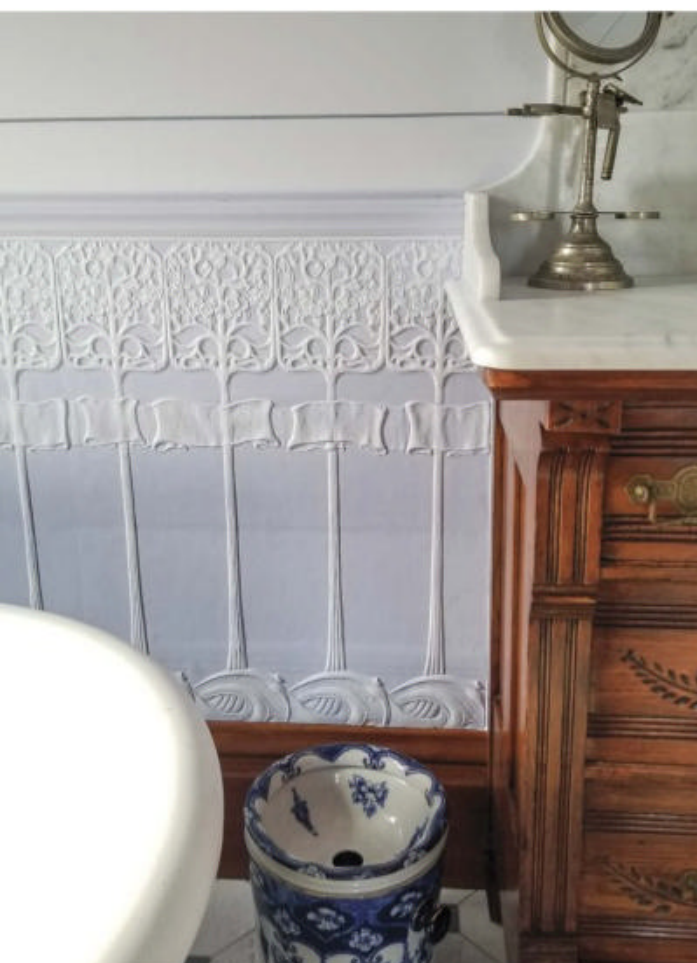
ABOVE The owner pre-cut each panel in the Lincrusta dado, carefully trimming the material to fit around moulded edges at windowsills, baseboards, and other wooden wall ornament. TOP RIGHT This once was the only bathroom in the 1895 Queen Anne house. Plaster walls and the floor had to go but the tub, toilet, and sash window were saved. Vaulting the ceiling made the small bath feel more spacious. OPPOSITE The narrow space between vanity and door allowed just enough room for an ornate Eastlake pier mirror along the wall.
