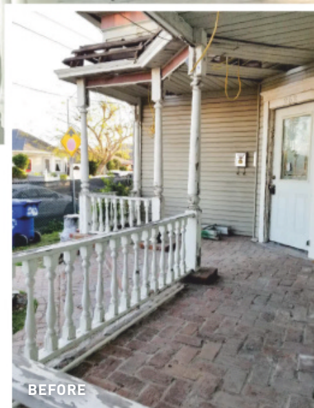
RIGHT The brick floor and ceiling of the side porch were damaged beyond repair, as was the gallery above. Most of the posts and balusters were worth saving. ABOVE The fully restored side porch with railings supported by original balusters. The homeowner had the porch ceiling painted the traditional, light "haint" blue.
