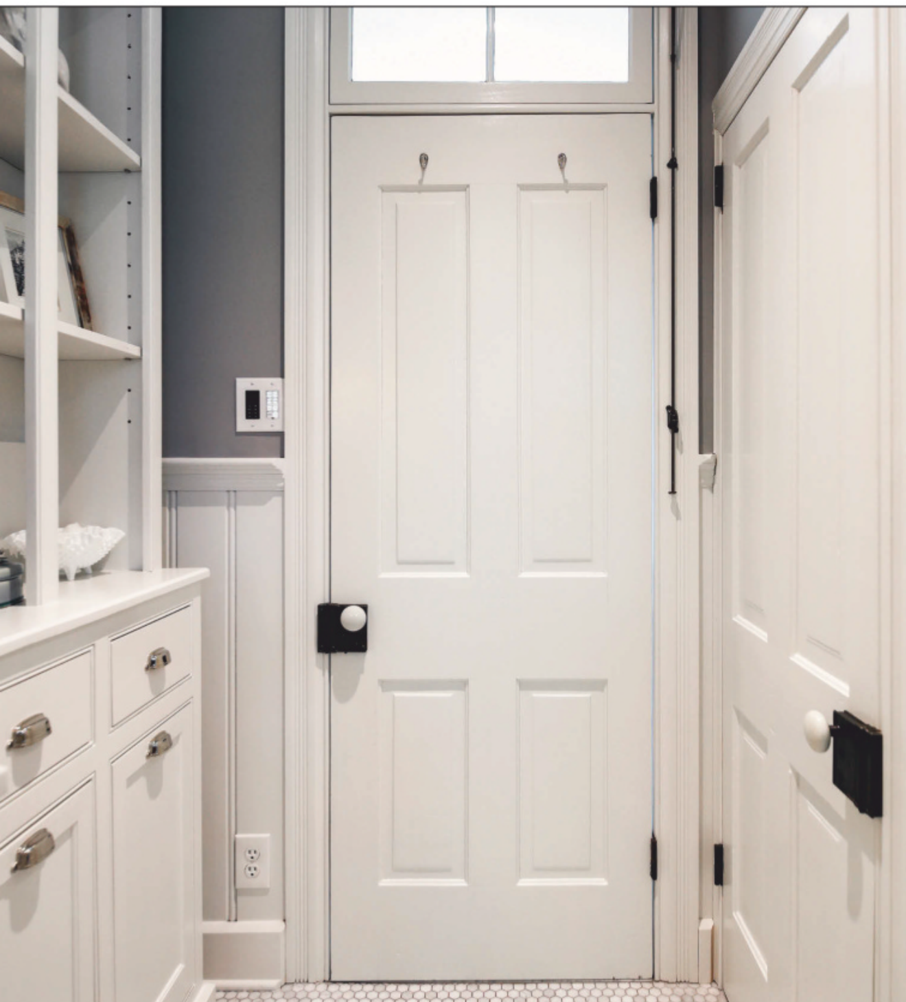
ABOVE In the Santantonios' finished bathroom, salvaged and restored rim locks with vintage doorknobs—and an iron operator for the working transom window—make the room feel original to the 1880s house.
