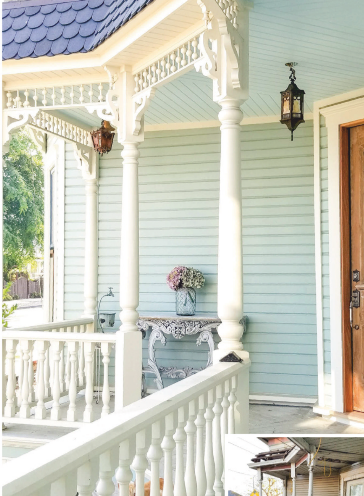
RIGHT The brick floor and ceiling of the side porch were damaged beyond repair, as was the gallery above. Most of the posts and balusters were worth saving. ABOVE The fully restored side porch with railings supported by original balusters. The homeowner had the porch ceiling painted the traditional, light "haint" blue.
