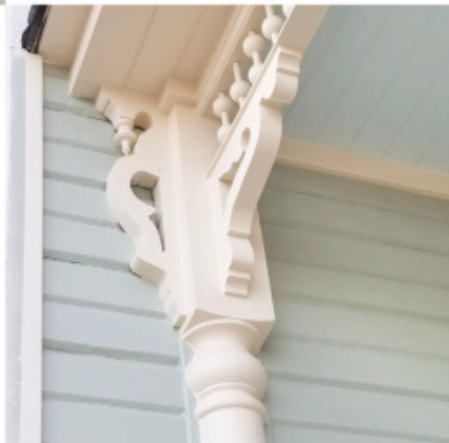
LEFT Scott Root of Abaroot Woodturning used salvaged wood to re-create the top of a post for the 1895 house, then hand-cut brackets. Spandrels came from Vintage Woodworks.
