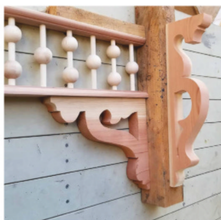
RIGHT One of the restored posts, with new brackets and the spandrel in place, on the finished porch.
