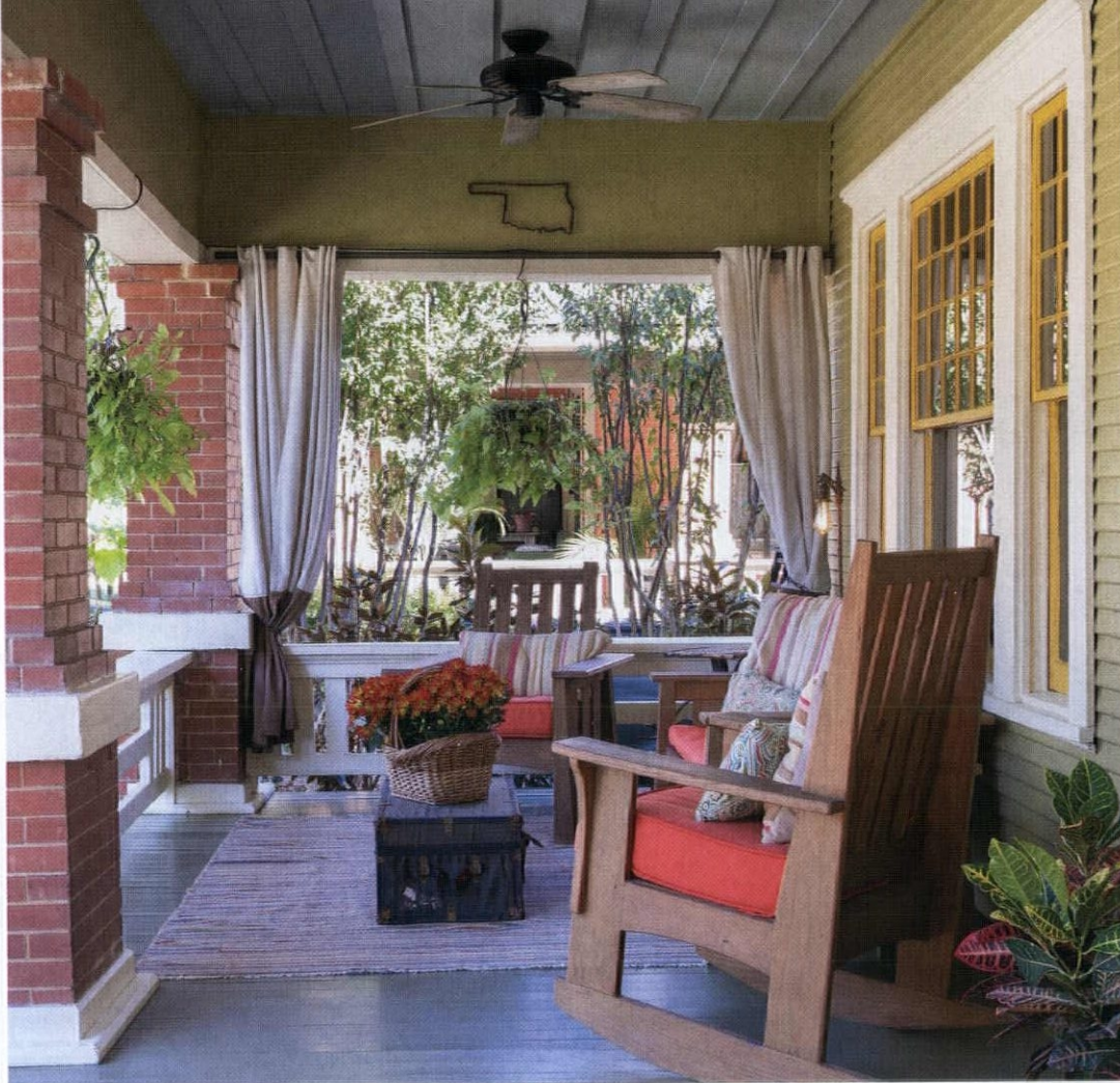
ABOVE Low wood balustrades span between brick piers in this variant of the Wilson-plan porch. RIGHT Vintage pillows decorate the reissued Harvey Ellis bed from Stickley. The rug was is by a contemporary Scots artist in the style of C. R. Mackintosh. OPPOSITE A 1930s vanity base was restored with Art Deco-style nickel hardware, then mounted with a prewar drinking fountain salvaged from a courthouse.
