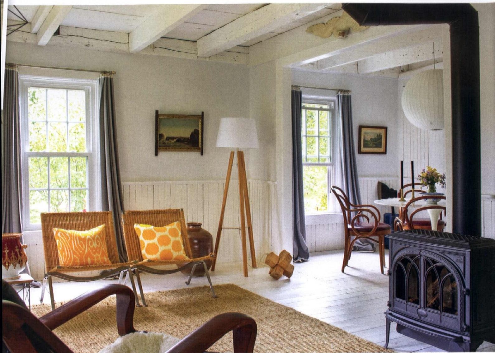
ABOVE In main rooms, acoustical tile and mid-19th-century plaster ceilings were removed to reveal the hand-hewn beams. Original wide-plank floors are pine.
