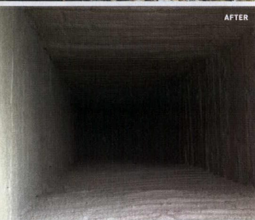
TOP Clay flue liners made by Superior Clay. LEFT An old square flue before lining; the same flue, after being lined using the Thermocrete process.
