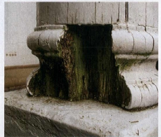
ABOVE An unvented wood column eventually rots from the inside.
