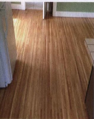
This custom floor involved cutting 2" boards down to 7/8", to match other floors in a 1920s house.
