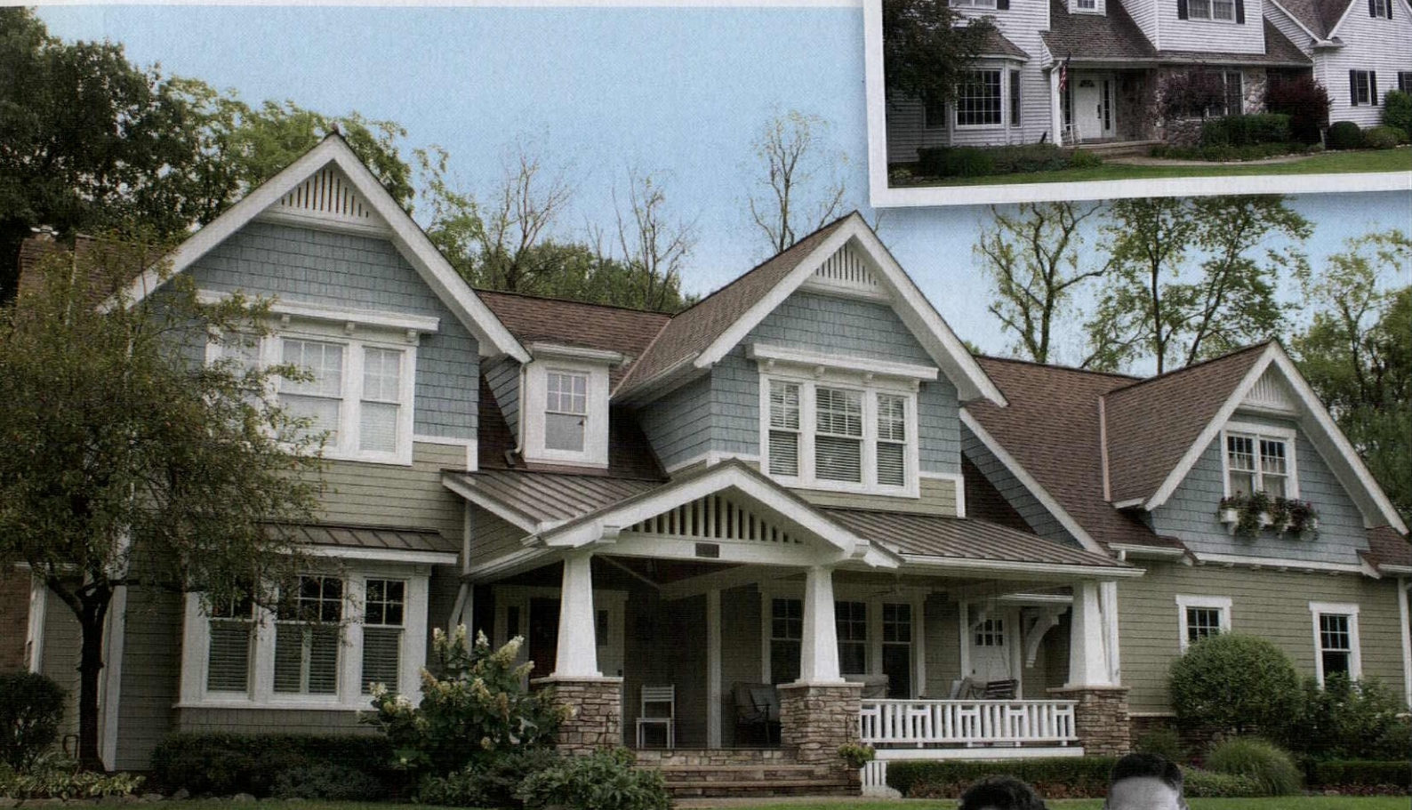
The makeover included new cladding and trim, a porch, and more proportionate windows.
