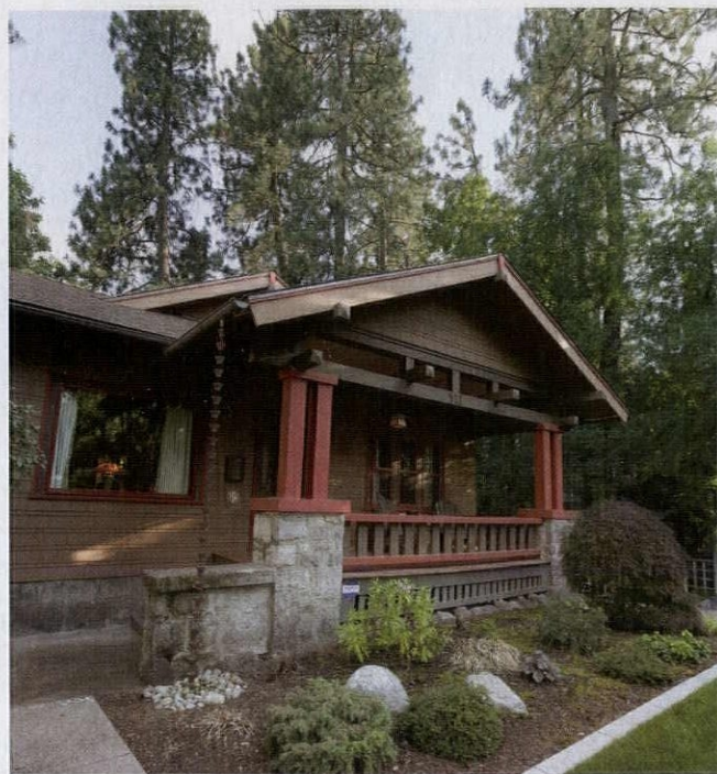
Early 20th-century charm was restored along with the front porch and a warm autumn color palette from Sherwin-Williams. New half-round gutters are held with spring clips, and a rain chain stands in place of a leader. Roofing is ‘Berkshire’ rectangular shingles from Owens Corning.
