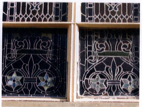
LEFT: Notice the bulging section, and missing and cracked glass in this 1890s staircase window. RIGHT: The bottom left side has been restored on this pair of 1890s panels. (Right side is before restoration.)
