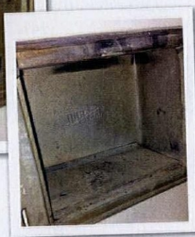
A MYSTERY: 1936 STEEL BOX IN AN EXTERIOR WALL, VENTED TO THE INSIDE.
