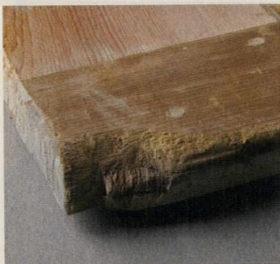
Damage to the lower corner and joint of this door (left) was repaired with patched-in new wood (right). This door will be painted, so the color of the replacement wood is not critical.
