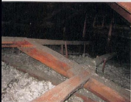
LEFT & ABOVE: In the attic above the kitchen ell are two previous roofs. The first (top) is fully intact and appears to date to the 1850s, while the shallower framing inside it (bottom) is likely pre-1820s.
