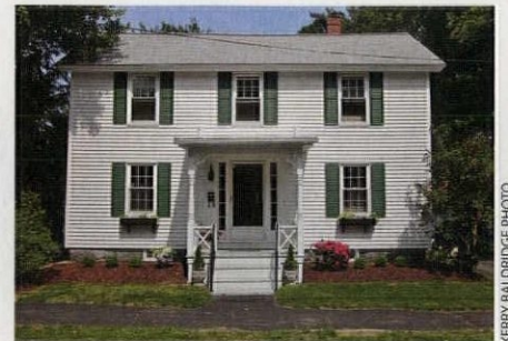
ABOVE: The Federal house in Exeter, New Hampshire, was augmented with a Victorian-style porch, likely in the 1860s.
