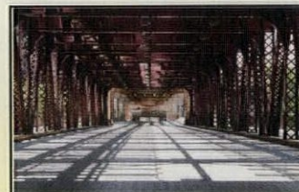
Heavy metal paint bridge restoration
