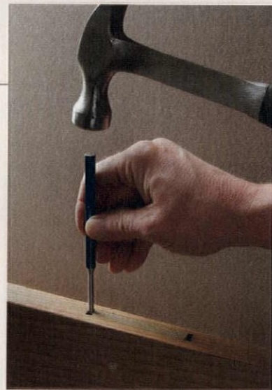
ABOVE: Tenon wedges often can be tapped in further or replaced with larger wedges to tighten joints. TOP: This door is out of square due to loose joints.
