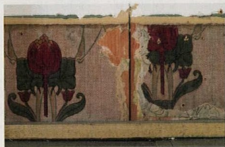
ABOVE: Inside this closet, Kerry discovered layer upon layer of wallpaper, including a pomegranate pattern underneath the trim (left) and a cream-and-white acanthus leaf pattern hidden beneath several layers of plaster (right).
