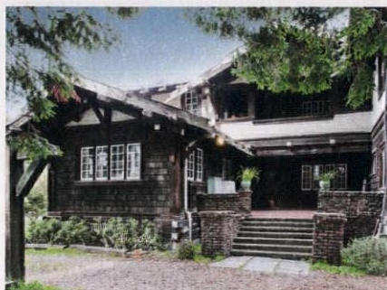
ABOVE: The 1905 Jesse Matteson House. OPPOSITE: The new layout placed the vintage stove and original kitchen dresser side-by-side.
