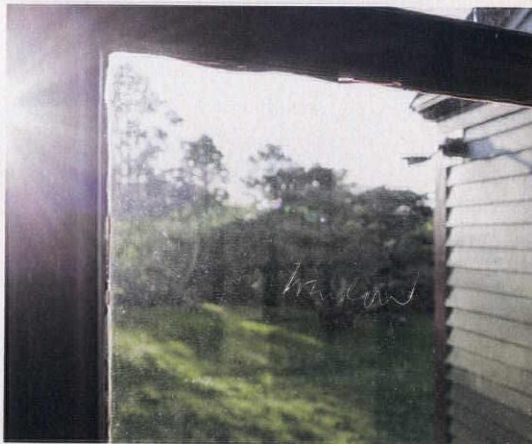
ABOVE: Before removing interior materials like beadboard and flooring (above), the team numbered individual pieces to make reinstallation easier. A pane of glass that the artist etched with his name (bottom) was carefully preserved.
