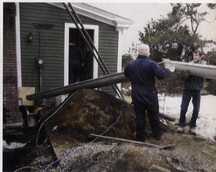
ABOVE: The team poured new concrete footings to stabilize the poorly constructed original stone foundation.
