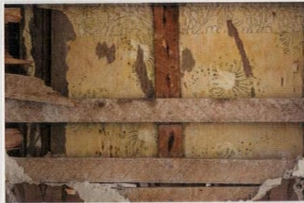
ABOVE: Inside this closet, Kerry discovered layer upon layer of wallpaper, including a pomegranate pattern underneath the trim (left) and a cream-and-white acanthus leaf pattern hidden beneath several layers of plaster (right).
