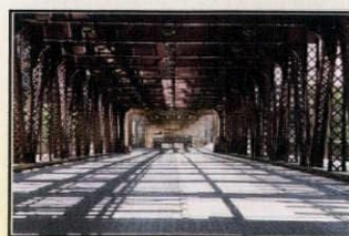
Heavy metal paint bridge restoration
