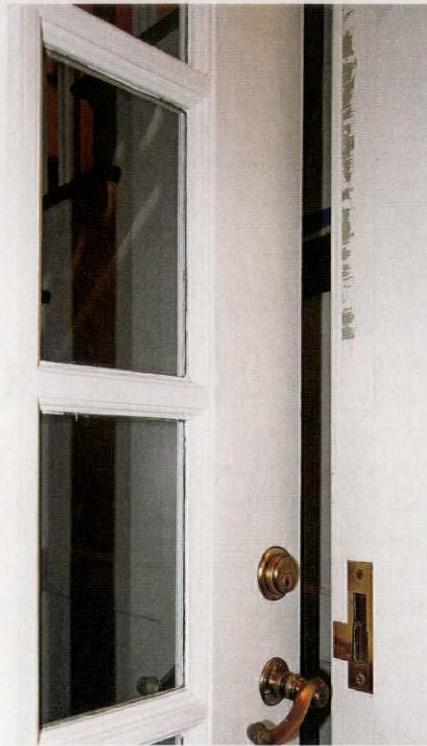
ABOVE: When doors aren't properly prepped before repainting, chips and dings are inevitable.
