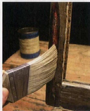
Deteriorated wood should be pre-treated, except in the few locations noted below.
