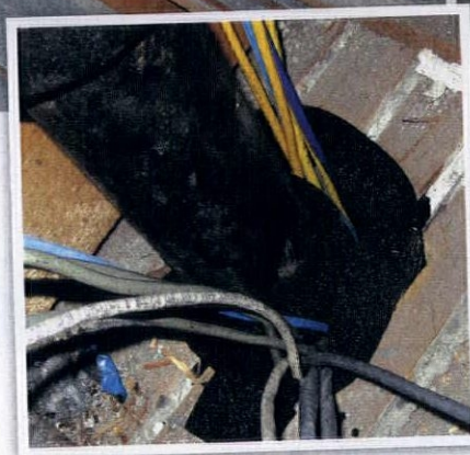
To help mitigate energy leaks, workers installed dense-pack cellulose in joist bays on the third floor (top left), insulated ductwork (above), and sealed penetrations around plumbing and wiring (left).
