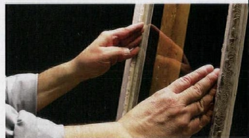
When placing glass, ensure the bottom edge rests on the lower glazing rabbet's neck.
