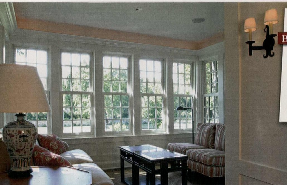
LEFT: The new sunroom's double-hung nine-over-nine windows allow for better ventilation than the previous fixed Plexiglas, which often caused the room to overheat. BOTTOM: A new built-in cabinet brought the study in line with the home's vintage architecture.
