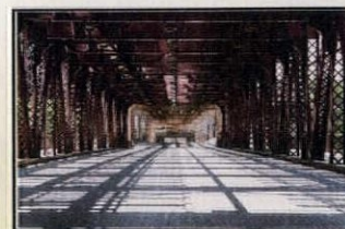
Heavy metal paint bridge restoration
