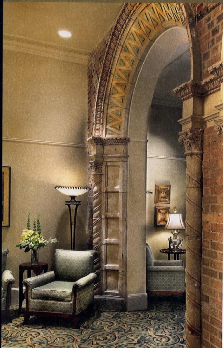
ABOVE, LEFT TO RIGHT: The hotel's façade was gutted and covered with a brick wall during one remodel; restoring it meant replicating original window trim. An original exterior wall was uncovered and restored near the ballroom. INSET: The hotel as it appeared in the 1930s.
