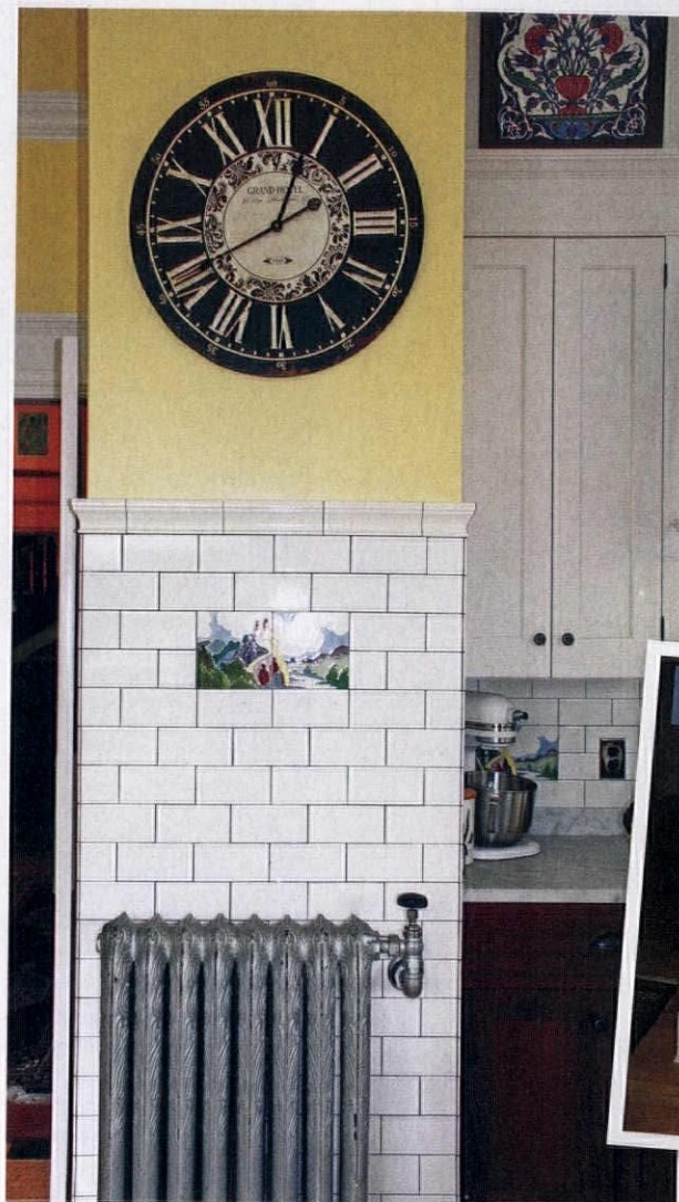
LEFT: In order to completely cover the walls in subway tiles, the radiator was removed, then re-installed. The use of white tiles with a dark grout helps to give the kitchen a French feel.
