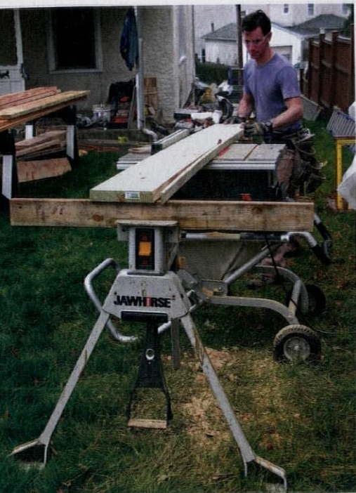
ABOVE: Outfeed support is critical for both production and safety, and enables you to work alone. Mark uses a 2x4 clamped to a Jawhorse to create a stable base. BELOW, LEFT: Mark made this work station using a sheet of plywood and some 2x4 blocks, all sitting on sawhorses bridged by 2x4s laid flat. Used to neatly organize tools, materials, and even coffee cups and cell phones, it keeps everything within easy reach, creating a tidy and efficient job site. BELOW, RIGHT: Portable table saws are best for ripping boards.
