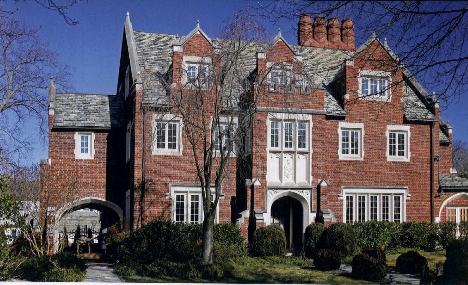
ABOVE: Old English designs are common; this formal Jacobean house features battlements, buttresses, and Tudor arches.
