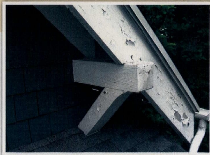
LEFT: The design of some decorative beam assemblies can become a water trap. BELOW: Solutions include (from left) replacing the beam entirely, splicing in a Dutchman patch, or filling the rotted beam with epoxy consolidant.
