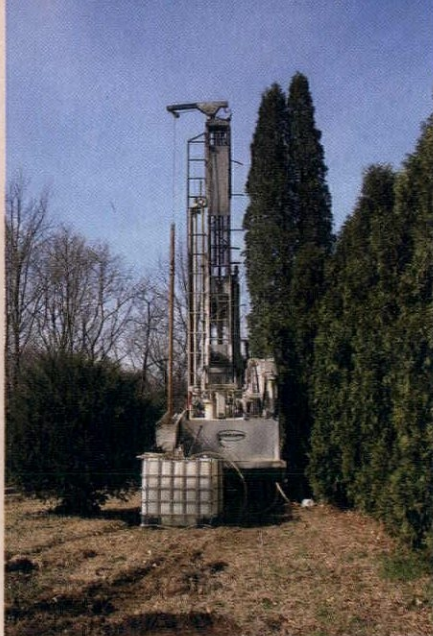
FROM LEFT: Installing the geothermal system first involved drilling six boreholes into the earth to access consistently warm temperatures. A trench between the bore field and the house holds both the refrigerant lines for the geothermal system and the electric wires for the solar array. Refrigerant lines in the attic run to the two separate units used to heat and cool the second and third floors.
