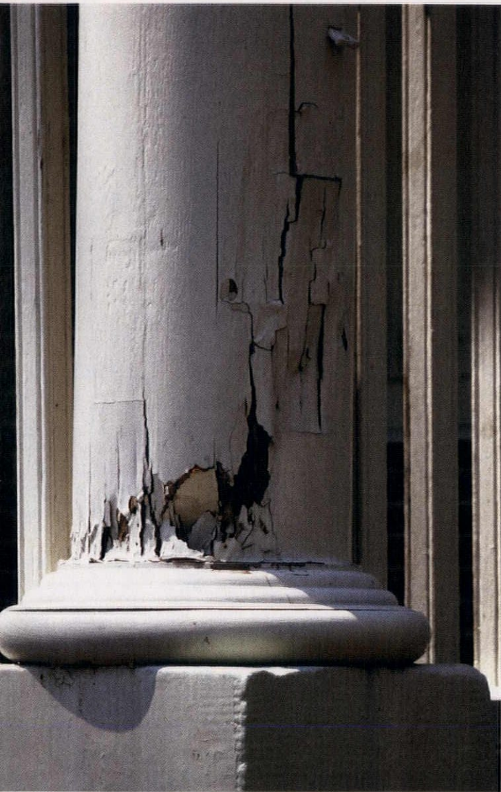
LEFT: Water seeping into hollow, unvented columns can create a breeding ground for mold; simple vents at the top and bottom of the column will allow water to evaporate.
