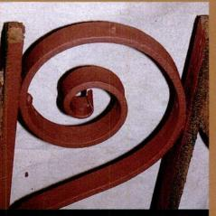
A good alkyd primer is critical, and should be applied as soon as possible after cleaning.
