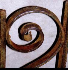
Iron that's been properly cleaned will be free of debris and ready for priming.
