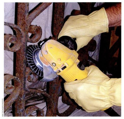
ABOVE: To make rusted iron good as new again, start by sanding away the corrosion—either by hand, or with the help of power tools (pictured). Use a light touch; you don't want to remove the intact metal beneath. BELOW: A hacksaw blade works well on crevices.
