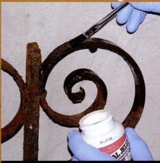
An application of Naval Jelly (without wire brushing) can work on lightly rusted iron.
