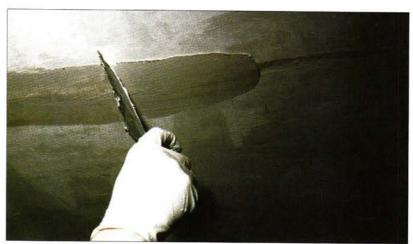
fill the crack, get your spray bottle again and thoroughly wet the V-notch, both inside and 3" on each side. This damp surface will let you remove buildup from your infill products.
