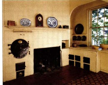
Above: To the left of the open hearth in the Rundlet-May House sits an original Rumford roaster. At the right is one version of his brick enclosed cooking range, which worked with specially designed pots.
