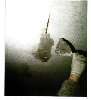
Above: Applying the first coat of compound from both sides to push it well into and under the crack. Right: Applying the second and third coats, the knife is held almost on end to scrape off excess.
