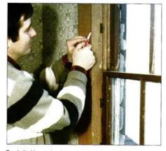
Far left: Use a hacksaw blade to cut hidden or stubborn nails. Large power-hacksaw blades (shown here) make ideal tools. Left: A good way to protect mouldings is to slip your pry bar between two wide-blade putty knives. Above: Before you begin prying, use a pen knife or wallboard knife to cut the paint and paper binding mouldings at joints.
