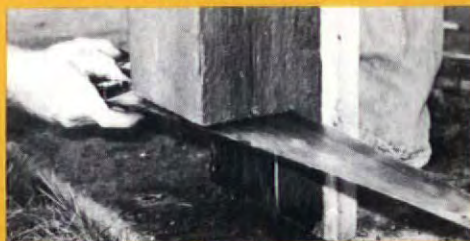
10" rotted bottoms of these load-bearing columns...
