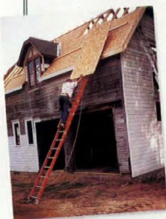
After we installed new sheathing and shingles, the building was dry for the first time in decades.
