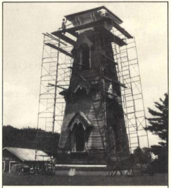
The extensive repairs necessary for the gingerbread, clapboards, etc., required full scaffolding to be set up.
