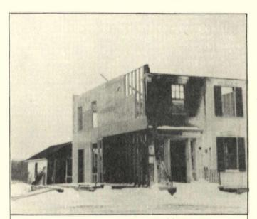
The house now shows the rebuilt portion, with the pediment removed for copying and salvage. The heavy bracing and studding is original.
