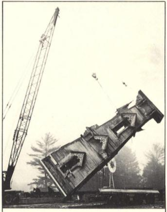
A 70-ft. crane raises tower onto its new foundation. For move, all projecting trim had been removed from one side.
