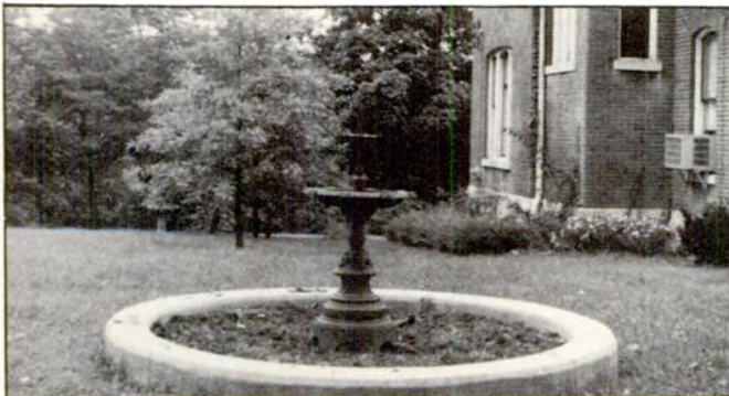
This fine example of a residential fountain is located in Anna, Illinois, and through repairs could run once more. It shows the typical cement basin that some of the iron fountains were constructed with.
