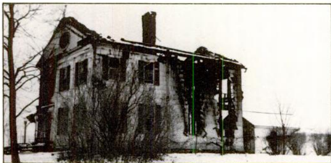
After the fire, not much more than the facade was left. All of the windows with the shutters remaining were saved.
