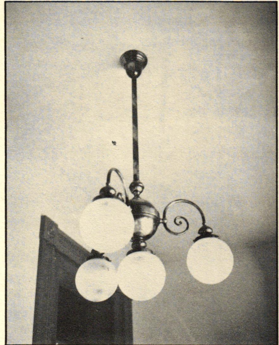
lighting with kerosene. Note the use of the reproductions of early electric bulbs—a must for proper restoration of a house museum but not a restoration for living. (2) This is an example of the oxidized early electric copper fixture. It came from an old house in Cape Girardeau. It is now in the pantry, added at the turn of the century, in the Glenn House. Notice the stripes.
