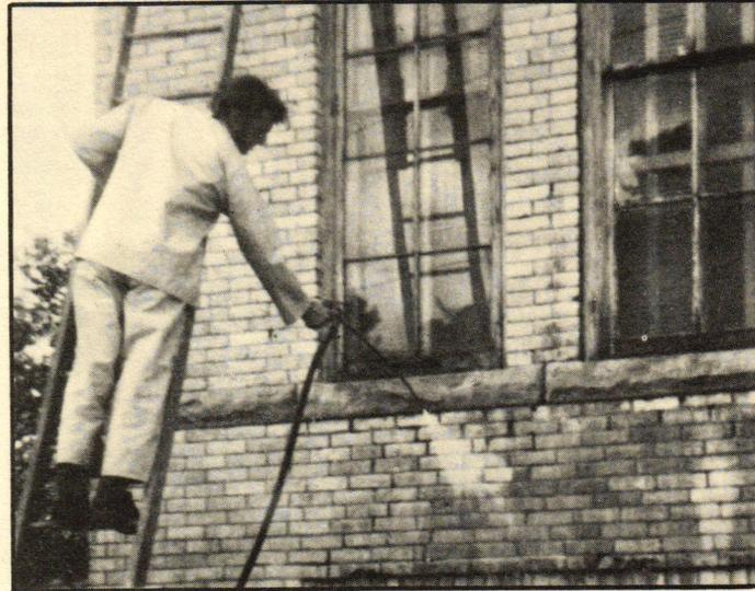
Thorough flushing of the brick cleaner requires a high-pressure (300-500 psi.) hose to remove all surface dirt. This equipment can be rented.
