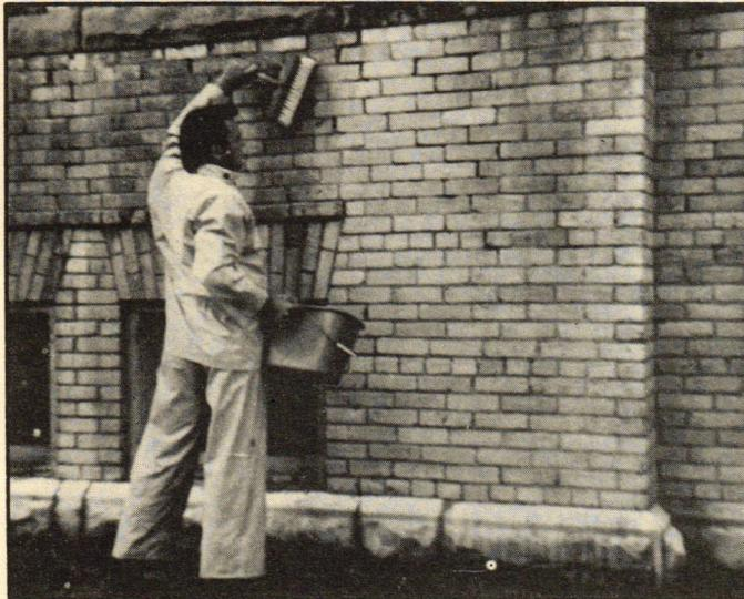
Acidic brick cleaner (which also serves as neutralizer for the caustic paint stripper) can be applied with a brush or ordinary garden sprayer.
