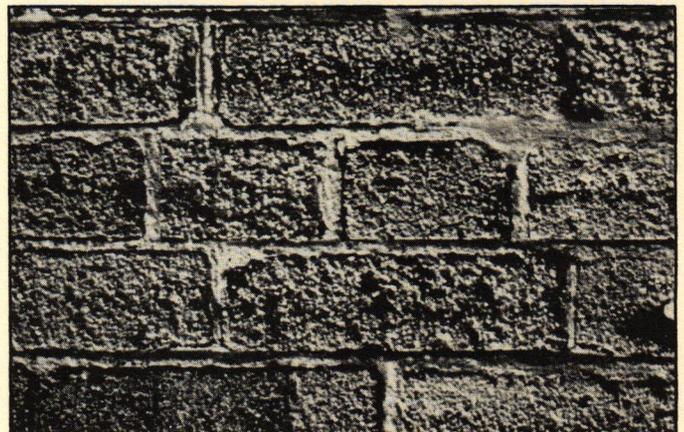
Sandblasting to remove paint can have disastrous results—as in this particularly horrible example from an 1890 brick church in Milwaukee.
