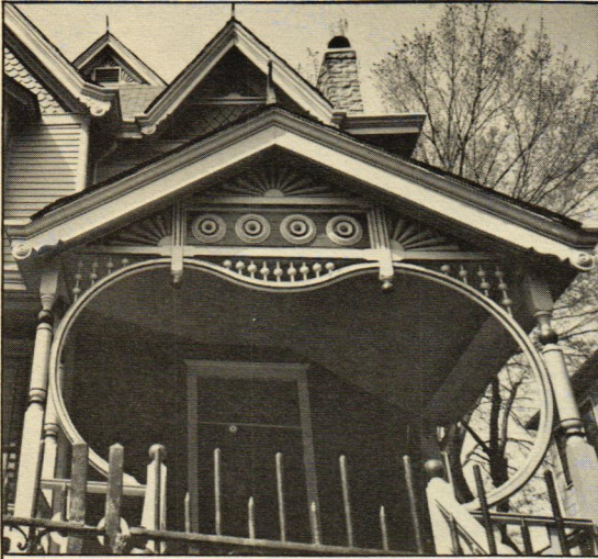
Porch, featuring Eastlake details, has had trim accurately restored. Exterior of the house has been repainted in the original Victorian red and brown color scheme.
