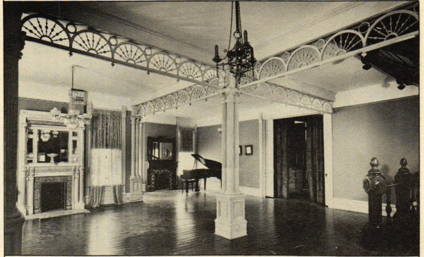
The 1,100 sq. ft. of space in the front parlors was probably used initially as a ballroom. The space is divided into quadrants by the overhead woodwork extending from the center column, all of which is painted ivory and gilded. One mantel is also ivory and gilt, two are cherry and the fourth is cypress.
