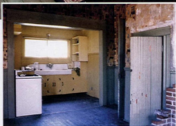
TOP: The place for dish storage and cleanup, the pantry has etched glass that was shipped from Liverpool (Roy's ancestral home). The Eastlake-style design was inspired by the staircase. This countertop is red oak. INSET: Site of the original pantry, before the 1980s renovation.
