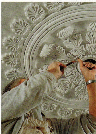
Artistic installations, such as this ceiling center by sculptor and master artisan David Flaherty, are done in plaster.
