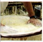
STEP 3: A layer of fine sisal fiber provides reinforcement. Fiber threads are stronger than woven fabric. Early plasterers knew this when they incorporated animal hair into plaster.
