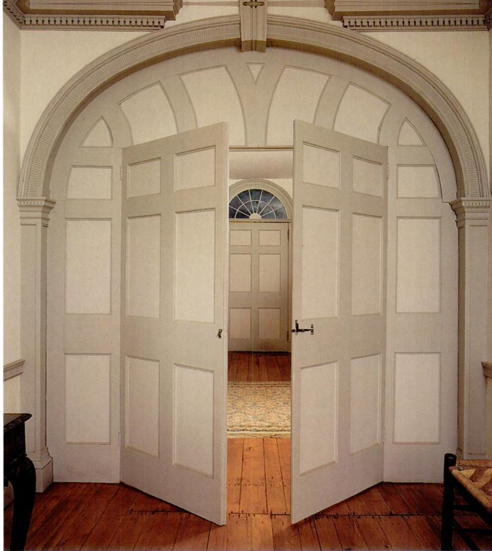
A historic paint scheme restores rightful emphasis to the exemplary late-Georgian woodwork of the Woodbridge House (1806) in the Berkshires of Massachusetts.
