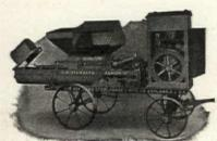
The measuring and proportioning of the cement, sand, gravel or crushed stone is done automat-
