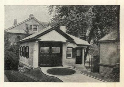
of the garage or smashing the top or guards will soon equal the cost of the turntable. The approach to the garage is not always a broad level stretch. Only too often there is a sharp turn or a steep grade with obstacles on one or both sides. A turntable is then the only stretched solution. practical solution.
