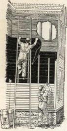
Architects, builders and carpenters of late years have been advocating the use of more advanced forms of insulation for walls, partitions, ceilings and floors-manufacturers of various so-called building papers and quilts have been put to the test. Even owners have pressed hard on the acquirement of an efficient lining for homes and buildings which should be in as far as possible, a non-conductor of heat, cold and sound. That is, that it should not allow those to pass through it.
