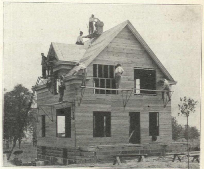
SHOWING ASHLAND FOLDING SCAFFOLD BRACKETS IN USE ON SIDES AND FOR CHIMNEY WORK.
