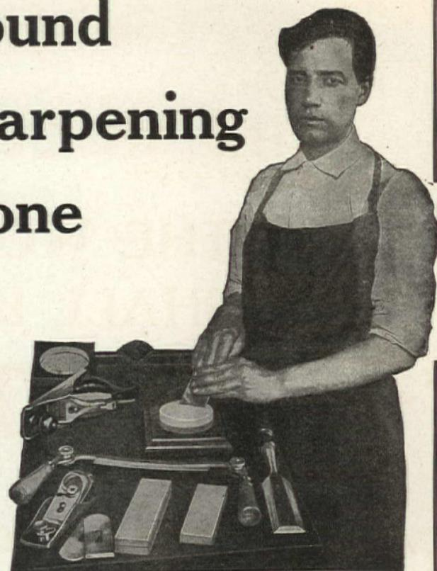
You can use the entire surface of the stone. You get the rotary motion so necessary in the sharpening of chisels, planer irons and so forth—and, as it is made of Carborundum you get the fastest cutting, most efficient sharpening stone on earth
