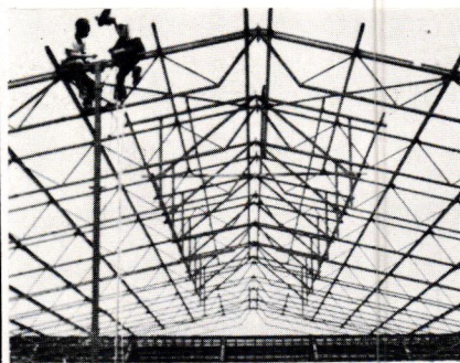
PORTAL FRAMES: Under construction in R.H.S. is this 120 ft. span 3 pinned portal frames — erected with light-weight lifting tackle.
