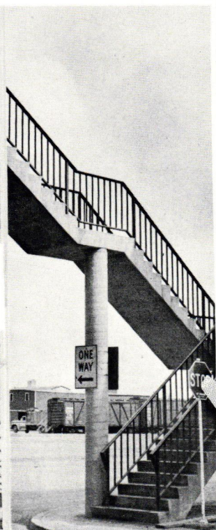
STAIRCASES: Here R.H.S. are used for handrailing on the staircase of a road over-pass.
