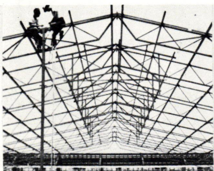
PORTAL FRAMES: Under construction in R.H.S. is this 120 ft. span 3 pinned portal frames — erected with light-weight lifting tackle.
