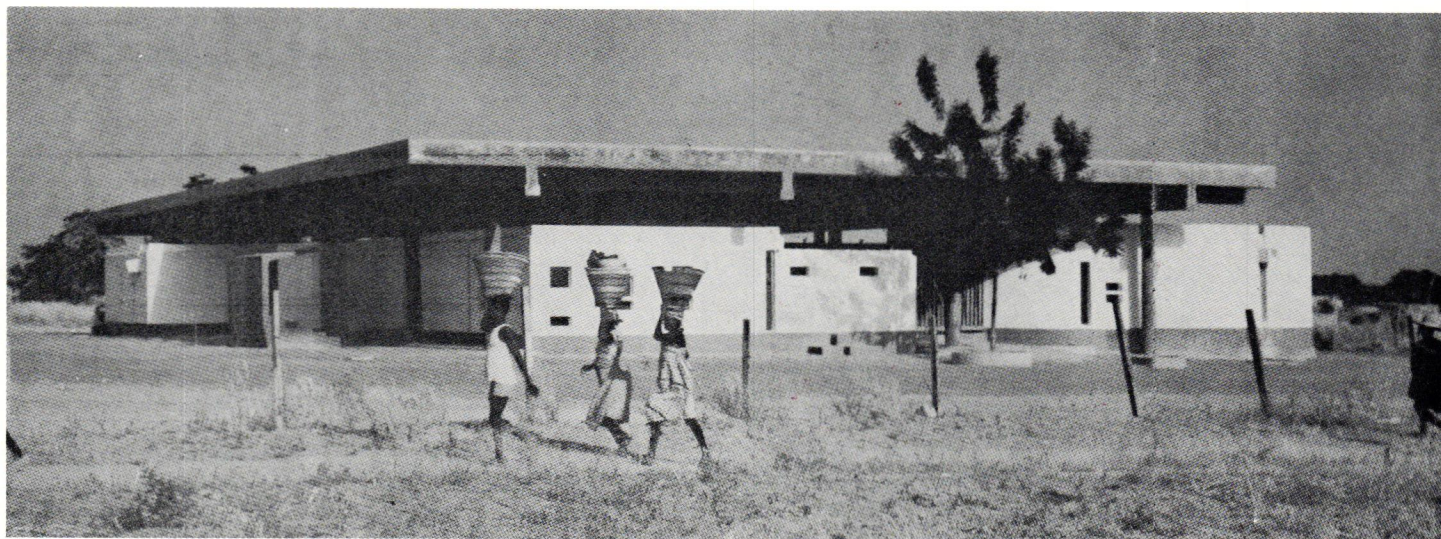
Above: The library consists of four separate buildings under a reinforced concrete 'umbrella'. There is a ventilating space between the underside of this roof and the tops of the buildings.
