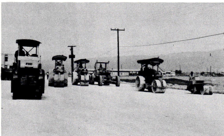
Preparing base for roadway — an essential part of the dramatic growth at Newport West.
