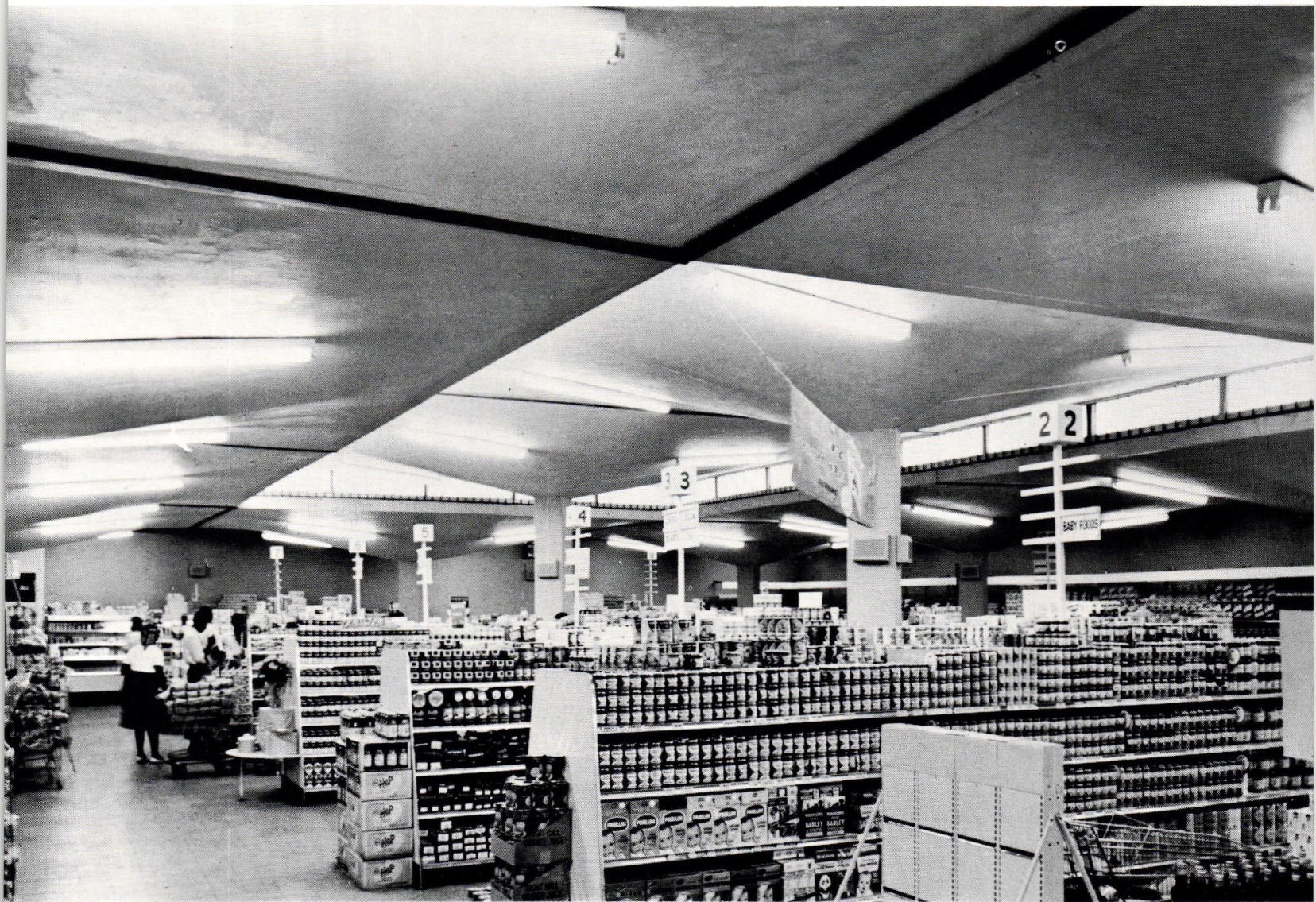
Interior of 'Stop-n-Shop' Supermarket—Showing HP Shell Roof
