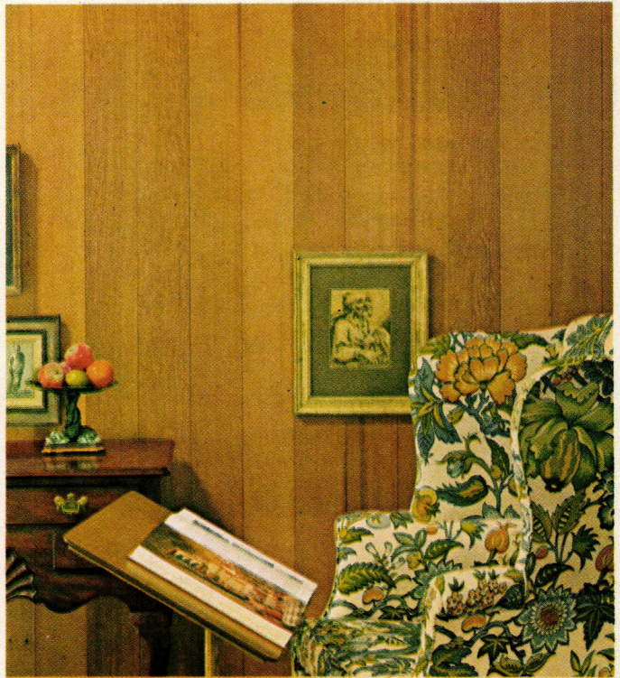
TONGUE & GROOVE pattern with a smooth face and narrow V-groove shows off the mixed grain of the redwood paneling.
