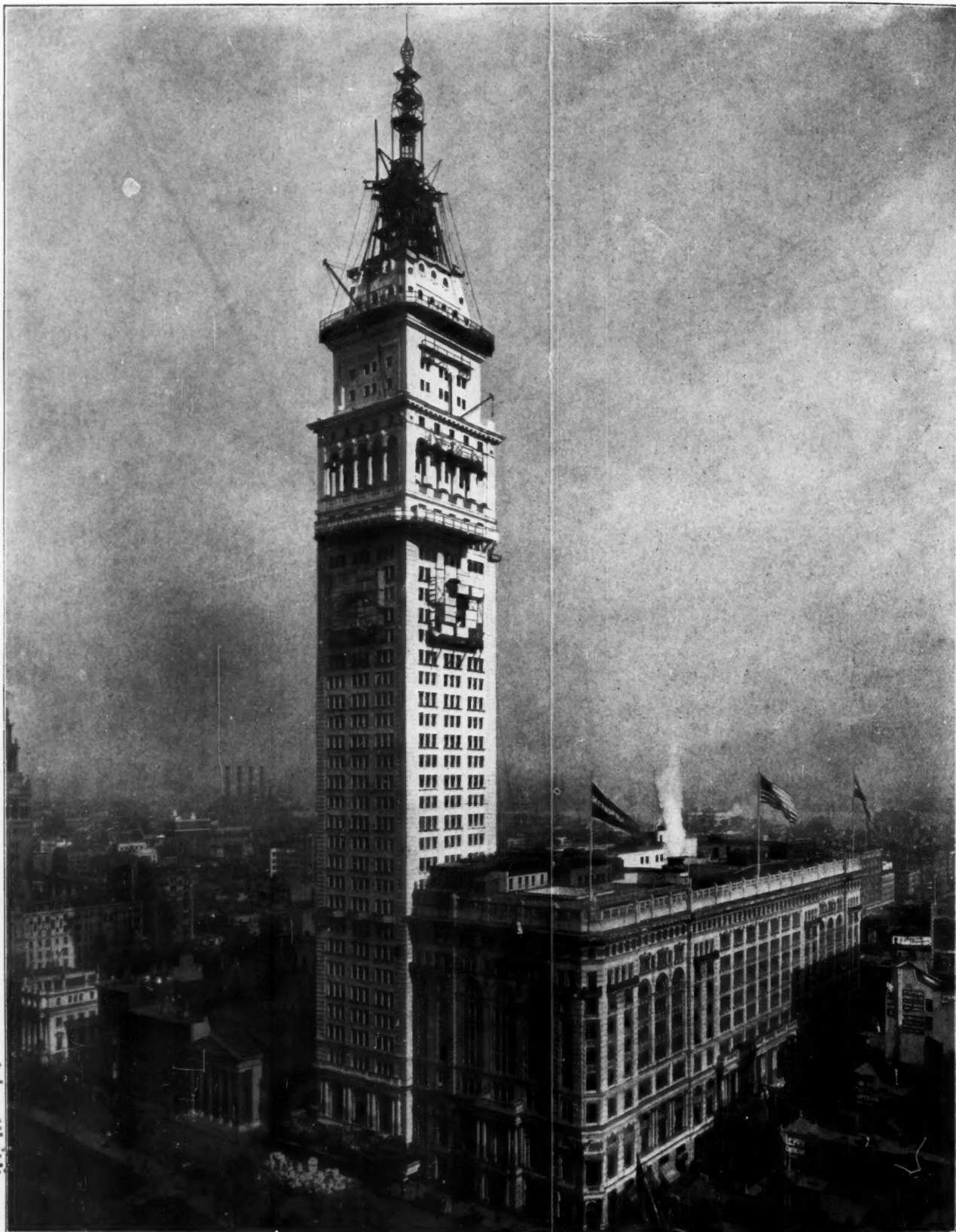
TOWER ADDITION METROPOLITAN LIFE BUILDING, NEW YORK N. LeBrun & Sons, Architects
