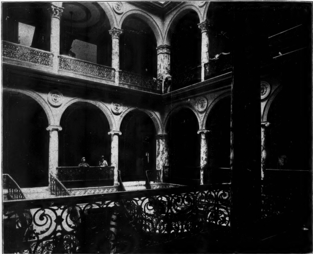
INTERIOR VIEW, ROCHESTER COURT HOUSE. J. FOSTER WARNER, ARCHITECT.
