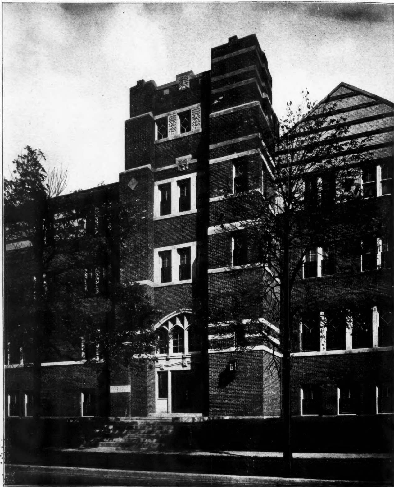
Detail of Tower
