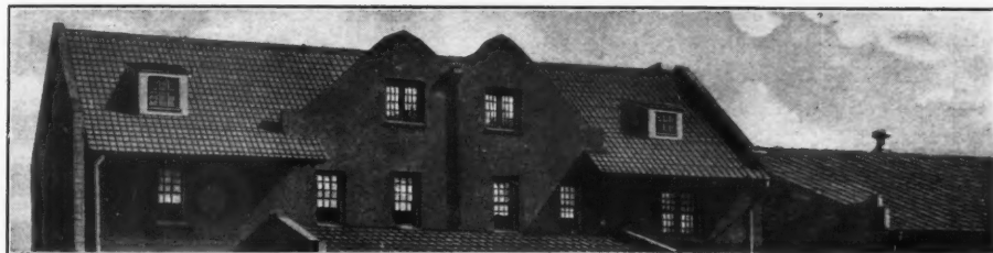
ASBESTOS "CENTURY" SHINGLE ROOFS—CLUB HOUSE AND OFFICES, PABST FARMS, OCONOMOWOC, WIS. Fernekes and Cramer, Architects, Milwaukee; Consolidated Sheet Metal Works, Roofing Contractors, Milwaukee
