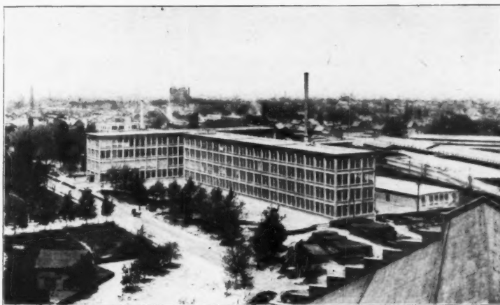
VIEW OF COMPLETED CONCRETE BUILDING.
