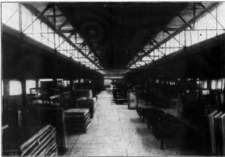
INTERIOR VIEW OF ONE-STORY BUILDING, SHOWING NATURAL LIGHTING, WITH LANTERN-ROOF CONSTRUCTION.
