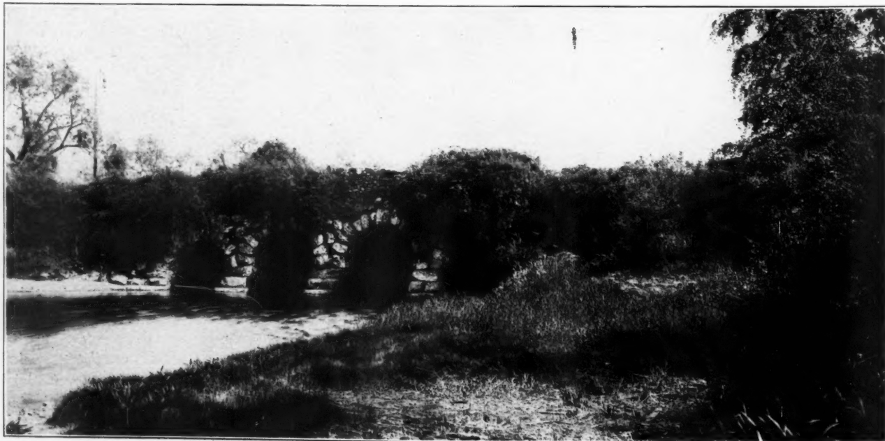
BRIDGE ON FENWAY.
