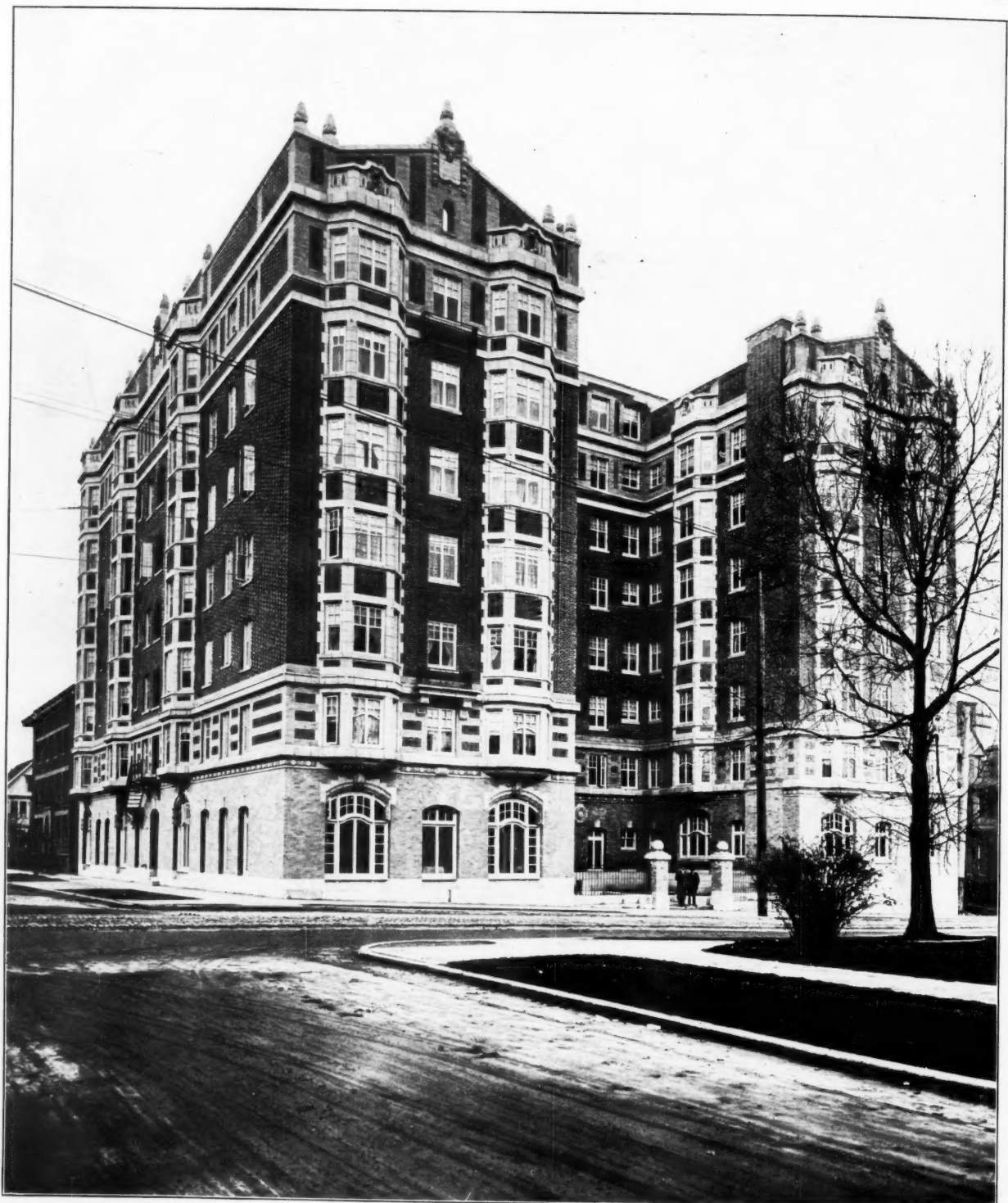
THE PERRY APARTMENT HOUSE, SEATTLE, WASH. Sommervell & Cote, Architects
