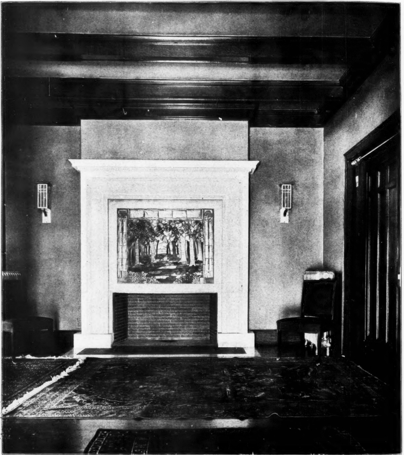
MANTEL IN HALL. HOUSE FOR E. J. MAGERSTADT, CHICAGO George W. Maher, Architect
