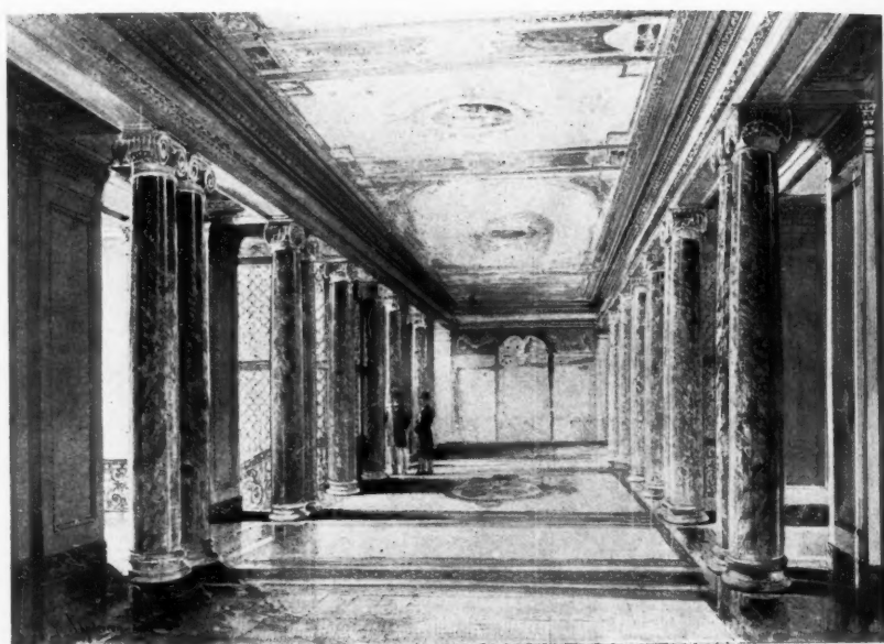
Interior View, Portland City Hall
