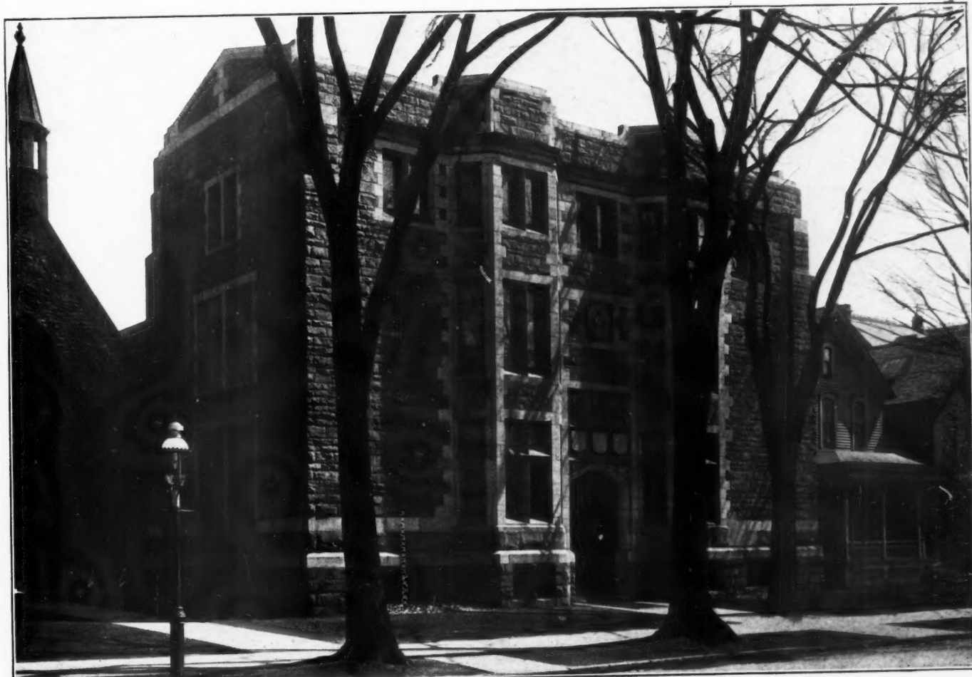
PARISH HOUSE OF TRINITY EPISCOPAL CHURCH. BUFFALO, N. Y. (Cram, Goodhue & Ferguson, Architects In Illustration of Article in this Number)
