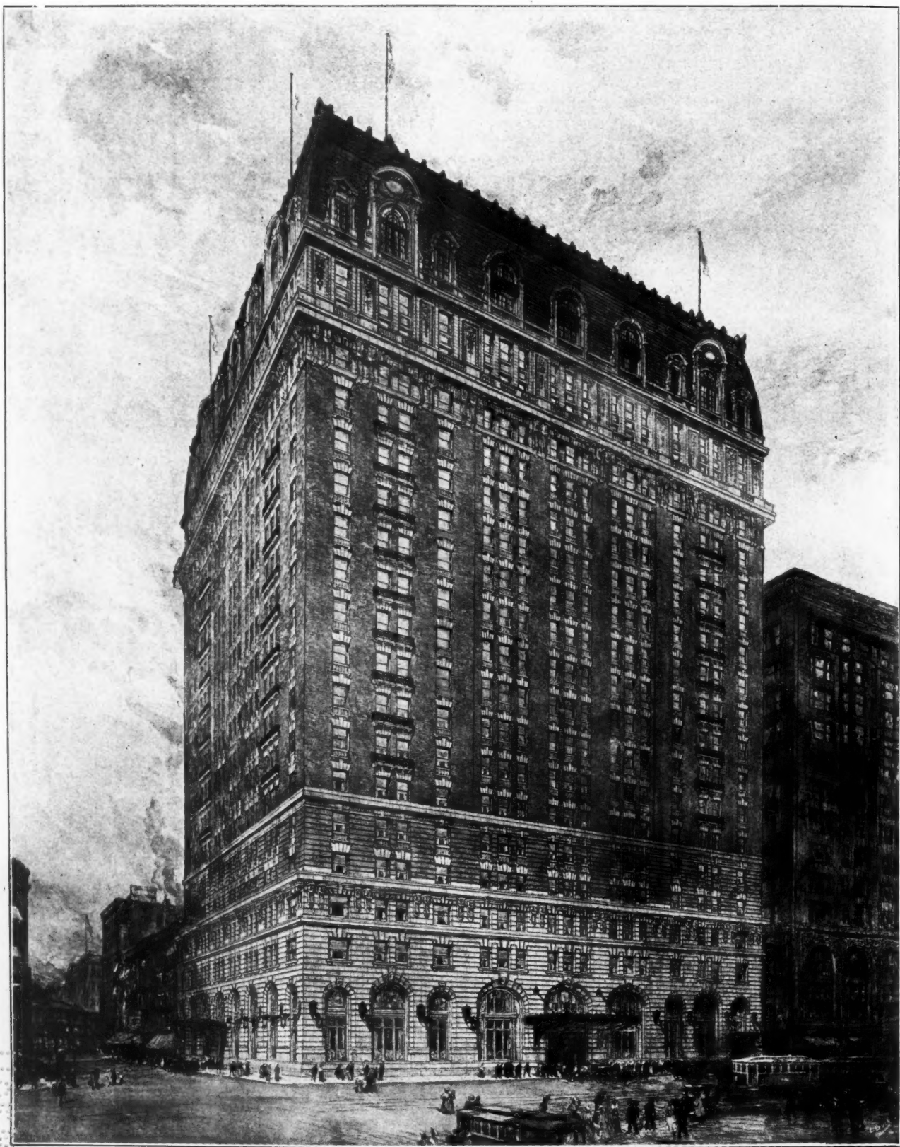
HOTEL LA SALLE, CHICAGO Holabird & Roche, Architects
