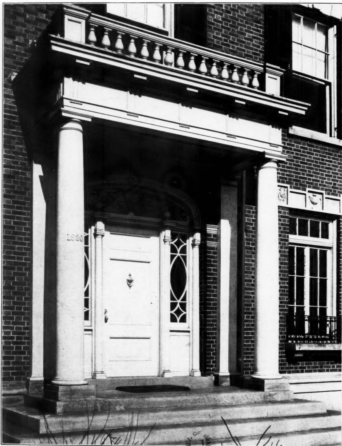
ENTRANCE DETAIL RESIDENCE OF MRS. F. J. GERAGHTY, CHICAGO Egan & Prindeville, Architects
