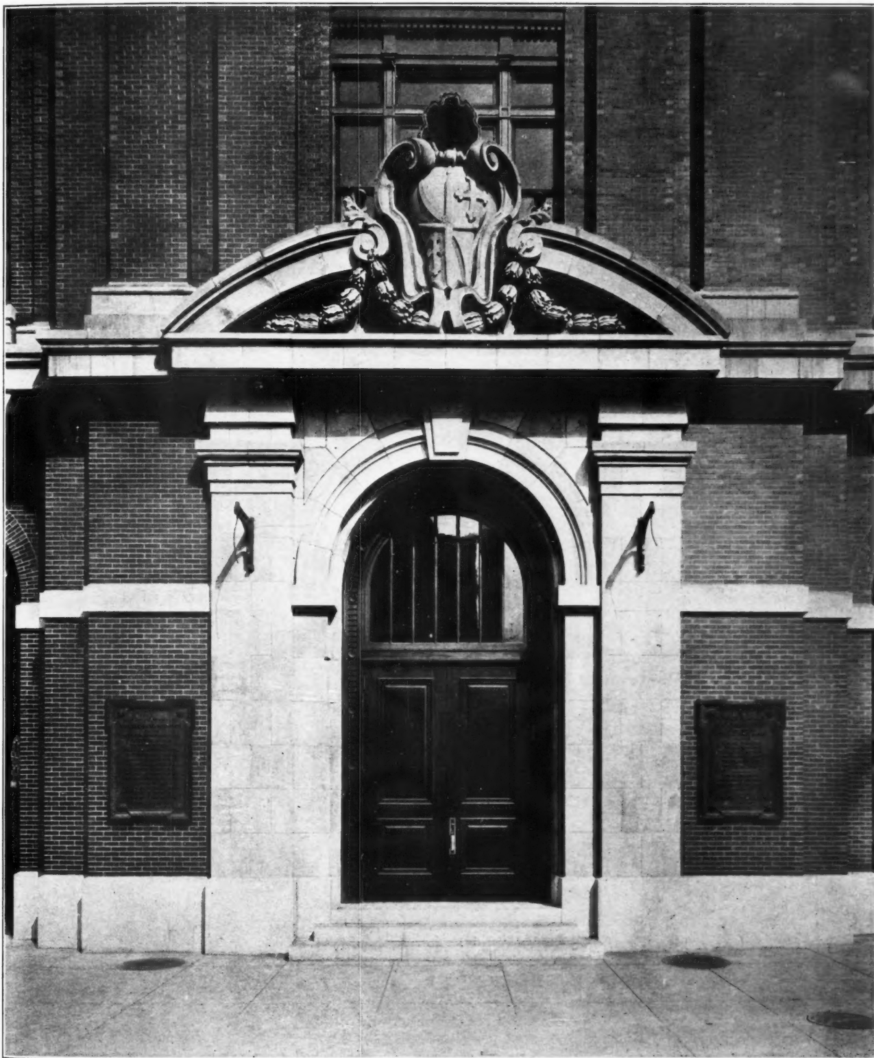
ENTRANCE DETAIL, MARYLAND INSTITUTE, BALTIMORE, MD.
