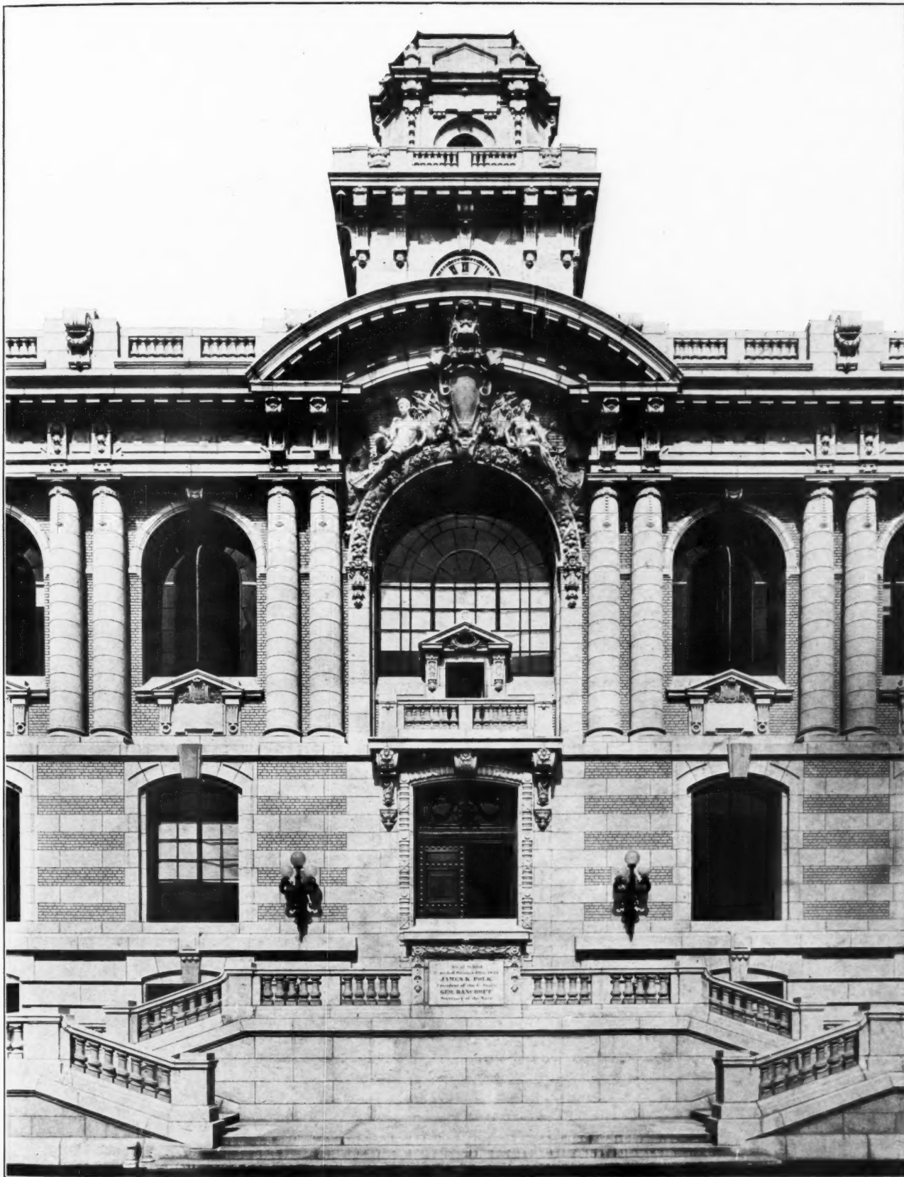
CENTRAL DETAIL. LIBRARY BUILDING. NAVAL ACADEMY. ANNAPOLIS. MD.
