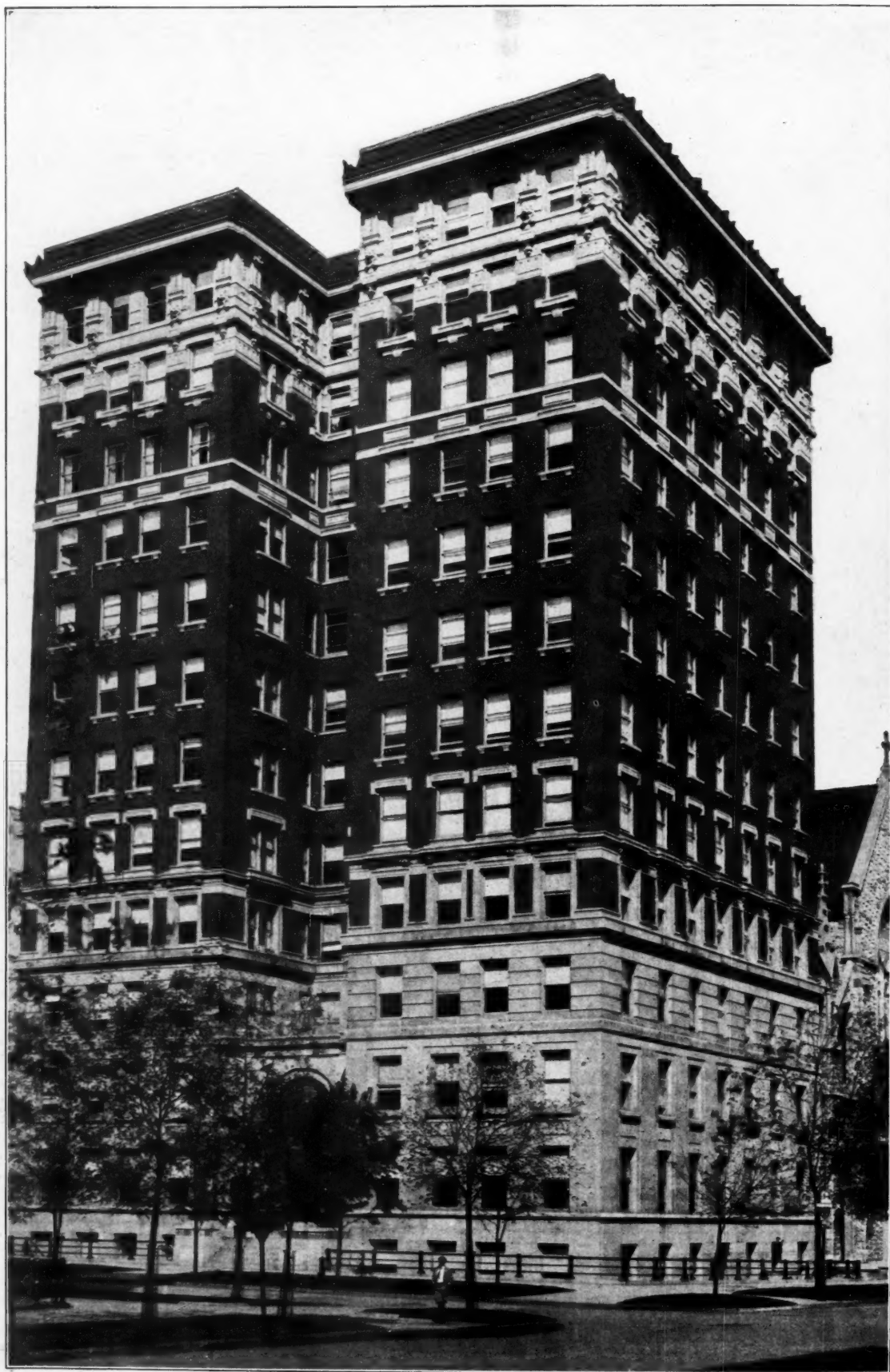
STANLEY COURT APARTMENT BUILDING, NEW YORK Charles E. Birge, Architect
