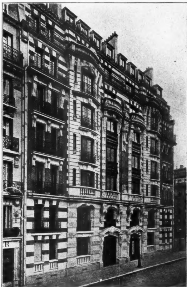
FIG. 13.—EXTERIOR OF APARTMENT HOUSE ON RUE CESAR FRANCE.
