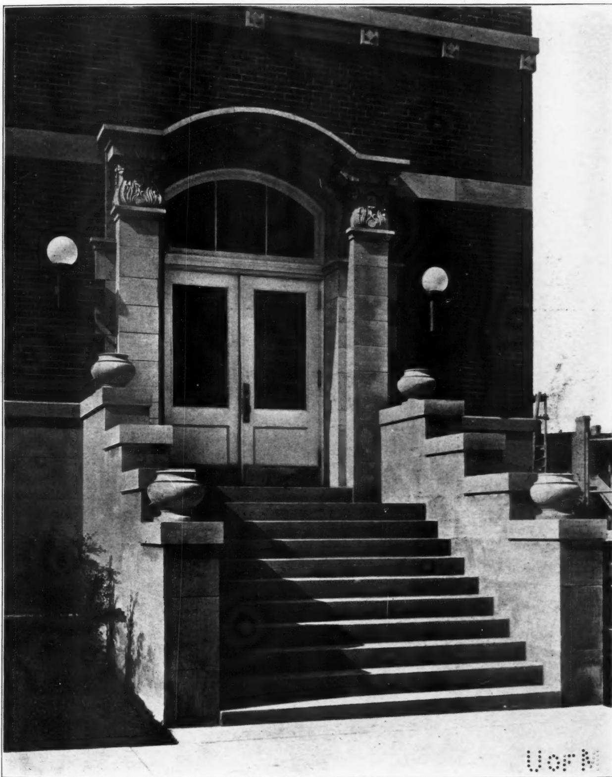
ENTRANCE DETAIL, EDGEWATER EXCHANGE, CHICAGO TELEPHONE COMPANY Pond & Pond, Architects
