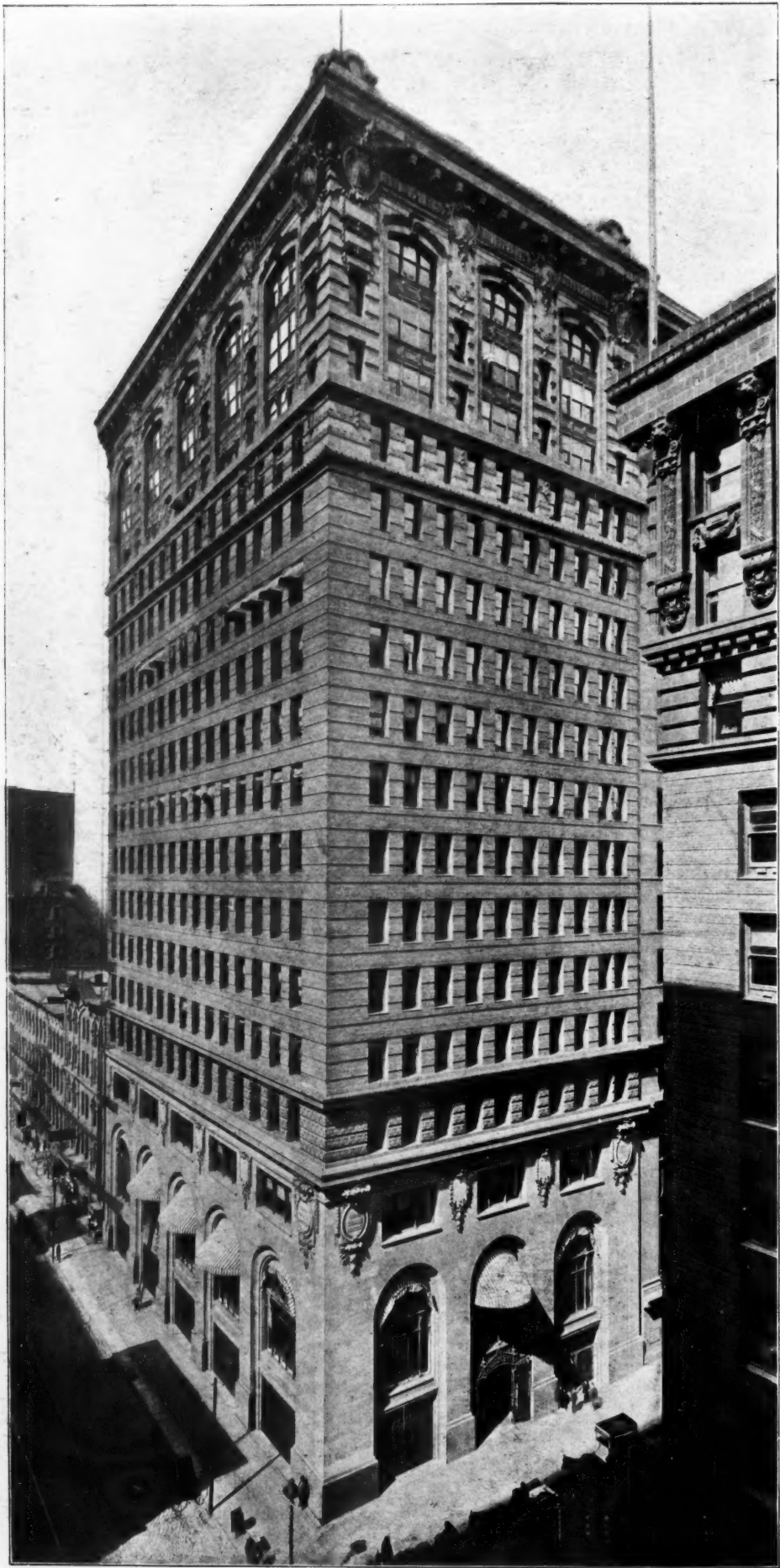
AMERICAN TRUST BUILDING, CHICAGO
