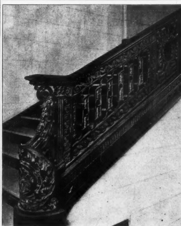
DETAIL OF RAILING, MAIN STAIRS UNITED ENGINEERING BUILDING, NEW YORK Hale & Rogers, Architects
